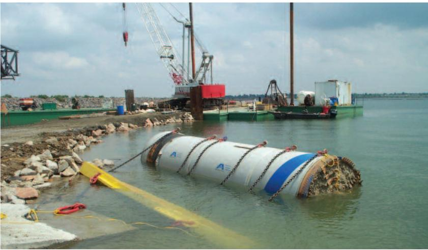
**Above:** The Akkerman MTBM about to be recovered by crane after the successful lake tap
