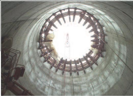
The Voest-Alpine roadheader in the 3.5m diameter, 293m long outlet tunnel
